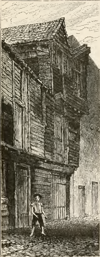
THE FIRST HOUSE SMITTEN BY THE PLAGUE. ASHLIN'S PLACE, DRURY LANE.
